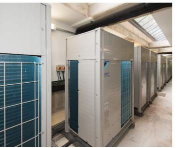
Overall control of the Daikin VRV IV systems is via iTouch Managers, with Power Proportional Distribution software and Bacnet gateway interfaces to the Building Management System. This facilitates accurate metering and billing, based on each apartment's energy usage.
