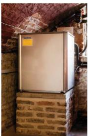
The Daikin Altherma HT system has a primary refrigerant circuit charged with R410A refrigerant. The hydrobox has Cascade technology - a secondary R134A circuit that produces the higher temperatures. The hydrobox also contains all the other necessary hydraulic components.
