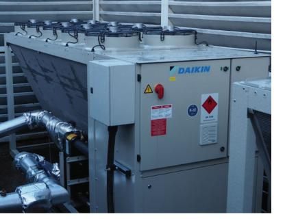
The EWAT-B units – Daikin's new generation of high efficiency air-cooled scroll chillers – improve seasonal energy efficiency ratios (SEER) by 10% in comparison with the previous R-410A range.
